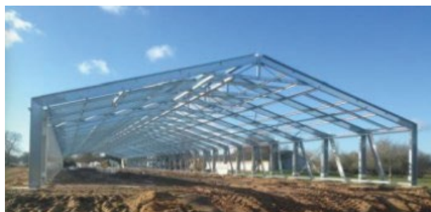
主钢架 C/H-section Main Frame Truss
