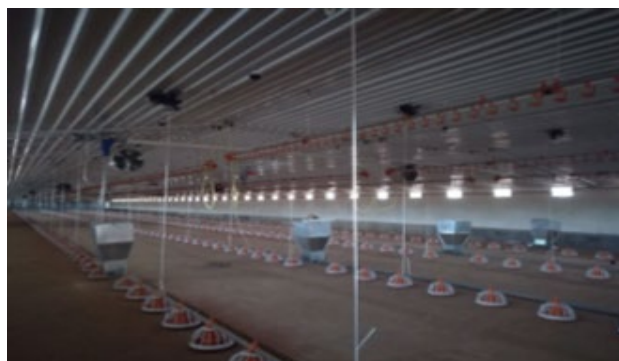
内部无钢架暴露 No main truss expose inside
